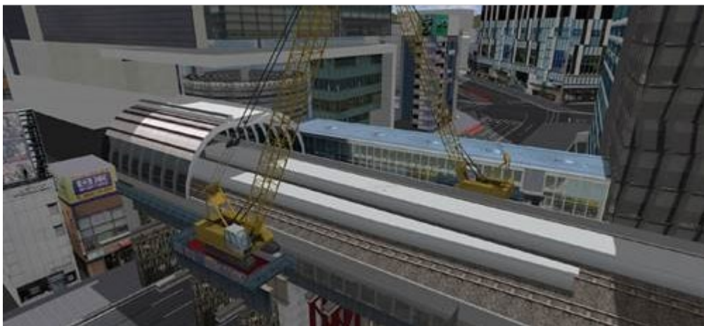
Simulation of the railway track replacement construction
